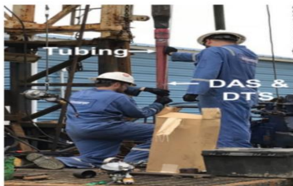
Fig 4: DTS being installed for Production and Injection Monitoring at Louisiana State University PERT Laboratory [2]
